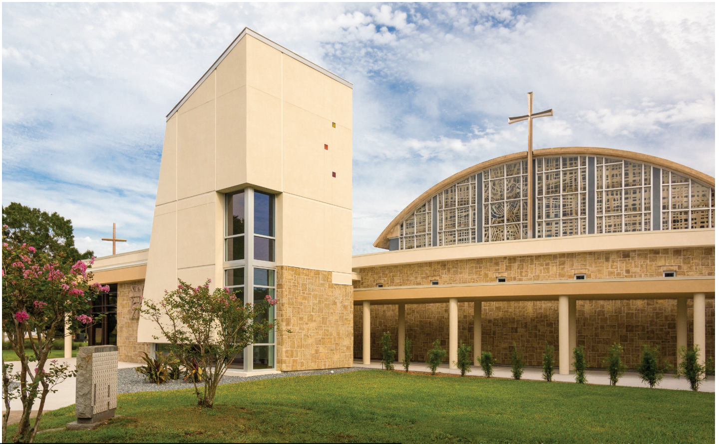
■ In 2015, the Prince of Peace Votive Church was renovated and serves as the National Shrine of Our Lady of La Leche at Mission Nombre de Dios.
